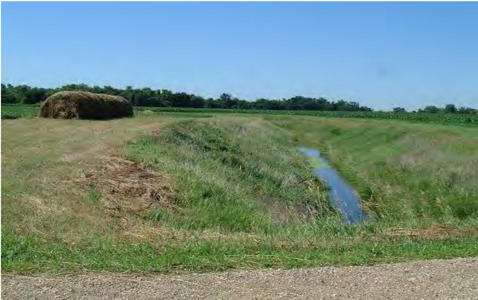
The board achieved completion of the enforcement of the 16.5 ft ditch berm law in 1999. From that time forward, each year, the staff completes a ditch berm inspection and reports back to the watershed on whether any ditch berms become out of compliance. Two ditch berms were reported out of compliance in 2009. Those landowners have been contacted and have indicated that they will reestablish the area to seed.
